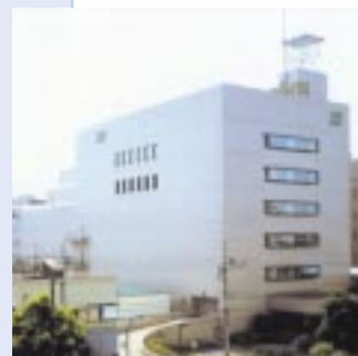
Tokyo Operation Center
